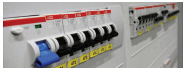
Figure 2.32 circuit breakers
