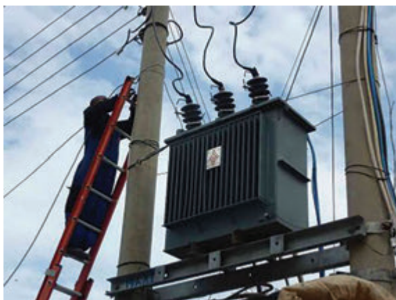
Figure 4.37(b) Roadside transformer
